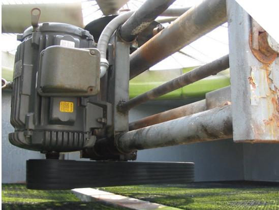
*Before: Cooling tower fan with 5 strand V-belt drive.*
