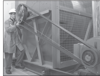
Using a string to check alignment
