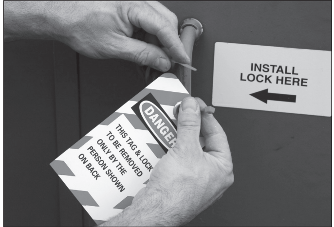
Turn off power, lock controls and tag
