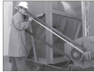
Using a straight edge to check alignment
