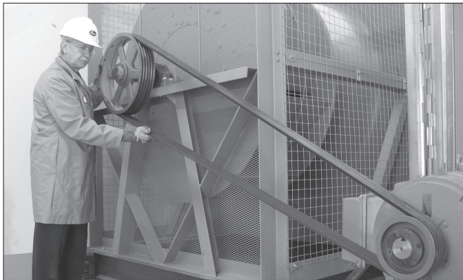
Begin by inspecting the belt
