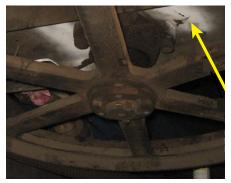
Beam cracked due to repeated shock loads during power up while unit was windmilling.
