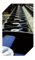
V-belts on 99 air-cooled heat exchangers at a refinery were converted to Poly Chain® GT® Carbon™ drives to eliminate slippage in hot weather. In addition to improved performance, the refinery realized annual energy savings of \$90,600 and an investment payback in less than one year.
